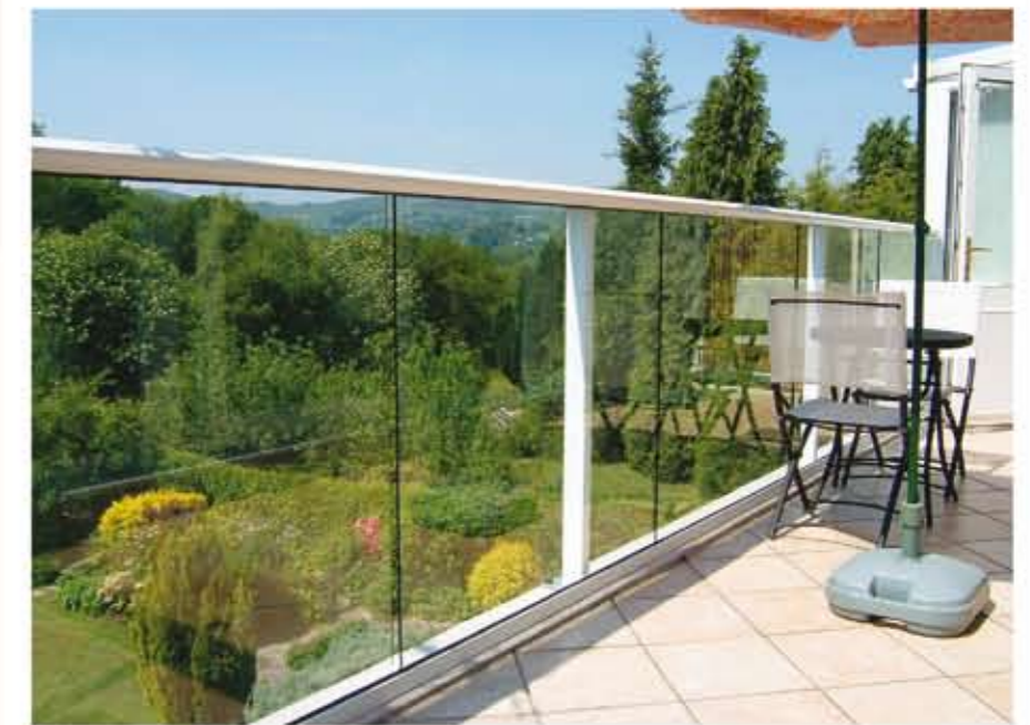
Balcony 2 System - handrail in white - Mold, Flintshire
