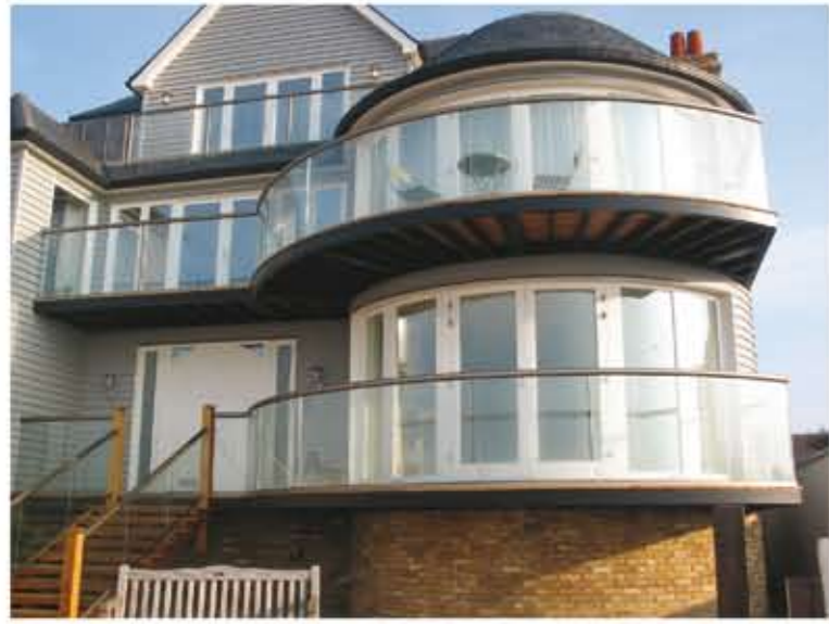
Balcony 1 System balustrades straight, curved and raked - handrails in bronze - Westgate-on-Sea, Kent
