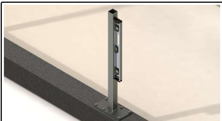
15) Position the primary post as per the drawings. Using appropriate fixings, fix the post(s) firmly to the structure making sure they are perfectly vertical.
