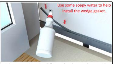
17) Once the silicone has fully cured replace the bottomrail clip bits with the full length glazing bead and wedge gasket. Trim off any excess gasket.
