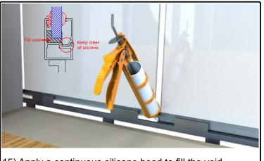
15) Apply a continuous silicone bead to fill the void between the bottomrail and the glass panel(s).
