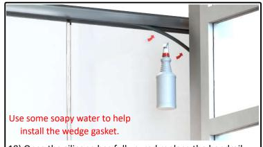
18) Once the silicone has fully cured replace the handrail clip bits with the full length glazing bead and wedge gasket. Trim off any excess gasket.
