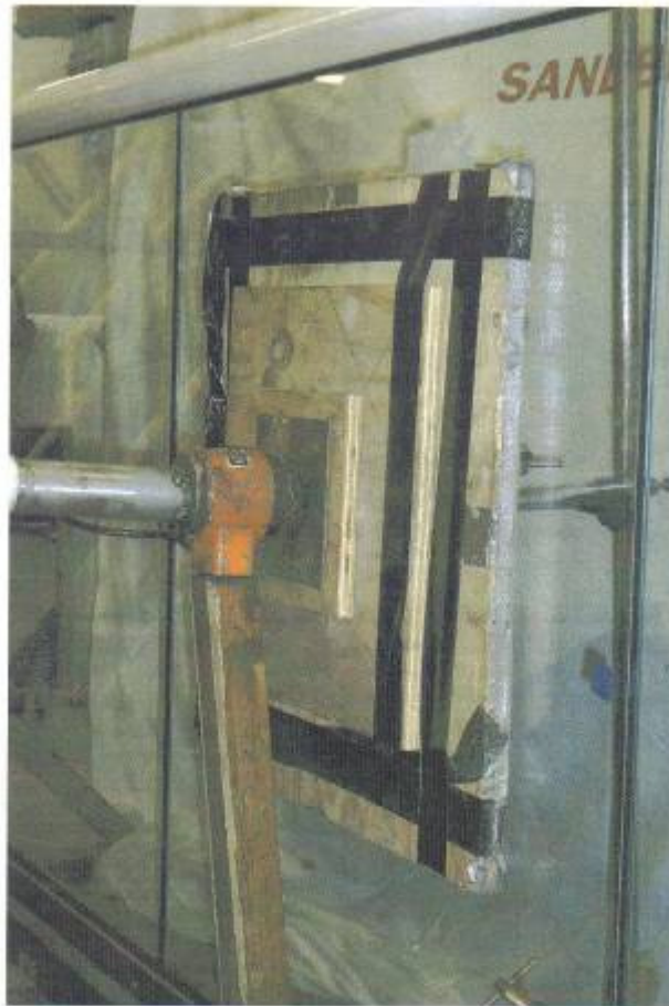
Plate No.4: Showing a close-up view of uniformly distributed test arrangement as applied to a central infill panel of the balustrade system.
